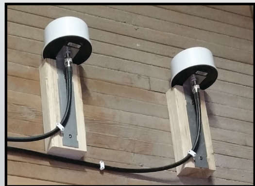
Two omni antennas using antenna hardware
