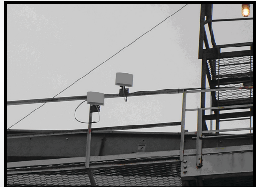
Two omni antennas using antenna hardware
