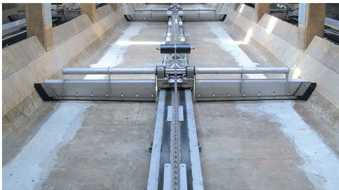
Clarifier Tank – Sludge Removal – Chain and Flight Drags
